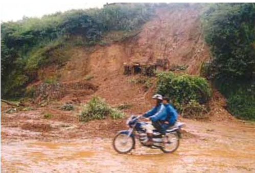
Figure 6. Flow-like landslide on roadside slopes of southern hills of Kathmandu, triggered by Rainfall of July 2002
